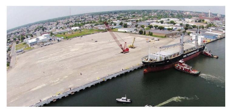
The New Bedford Marine Commerce Terminal is a multi-purpose facility designed to support the construction, assembly, and deployment of offshore wind projects, as well as handle bulk, break-bulk, container shipping and large specialty marine cargo. The first of its kind in North America, the terminal has been engineered to sustain mobile crane and storage loads that rival the highest load-bearing ports in the nation.
